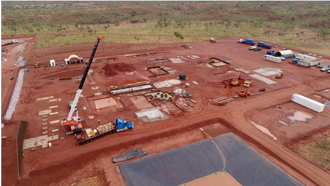
Concrete works advancing in Beneficiation and Hydromet areas
